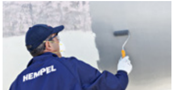
Apply Hempel's Underwater Primer onto prepared surface
