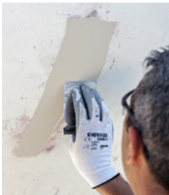
Fairing any defects
